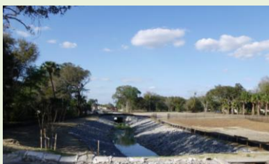
The stabilization project involved extensive use of recycled concrete serving as riprap to armor the creek bed and limit erosion.
