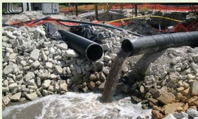
A gravity drain network overlaying recycled concrete was used to divert 500 feet of an onsite creek during remedy construction, which reduced use of diesel pumps.
